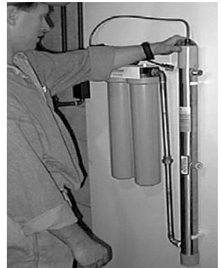
Installing UV unit
