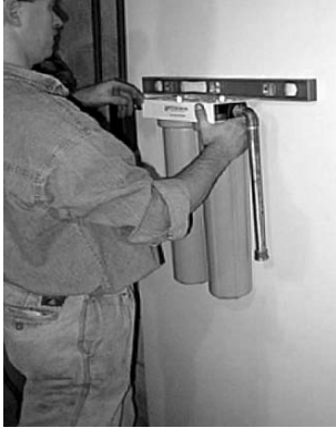
Installing UV unit
