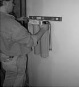
Installing Pre-Filter set
