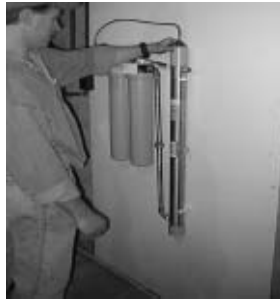
Installing the UV unit
